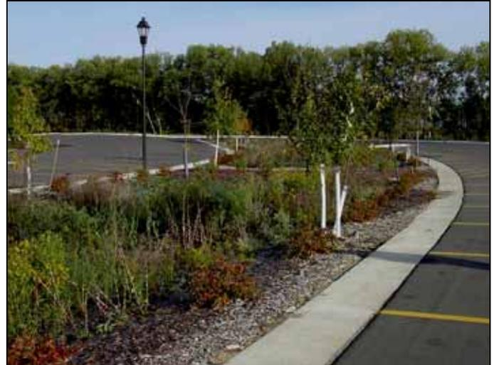
Restoration will address existing and new development. Above is an example of a vegetated swale that collects and treats stormwater from the surrounding parking area.
